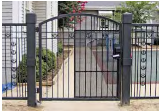
Dillard designed and installed gates for Grace-St. Luke's Episcopal School.
